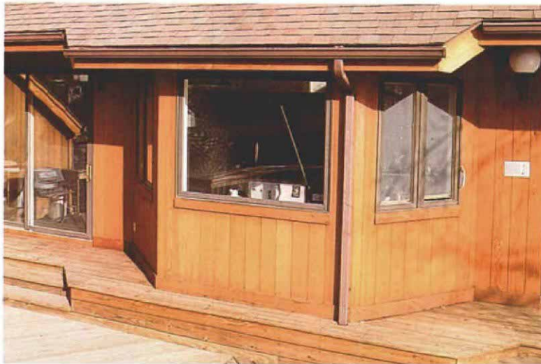
When an angled bay is capped by an extension of the main roof, the rafters that sit on the angled walls require some careful cuts.
