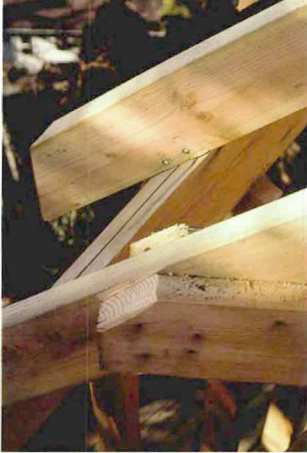
Method #4: beveled header/no bird's mouth. Here the header is beveled in plane with the bottom of the rafters. There is no need for bird's mouths; the rafters simply bear on the headers (above left) and are held in place by toenails. The bevel angle for this header was determined by the top of the gable-wall plate where the two intersect (above right). The bottom end of the header is recessed below the level eaves-wall plate.
