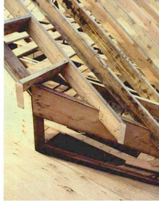
Method #5? From this view, you can't tell whether the header is notched for the rafter or vice versa. The author tried the former but thinks the latter method, which he tested on a model, might be the best
