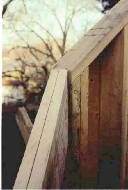
Method #4: beveled header/no bird's mouth. Here the header is beveled in plane with the bottom of the rafters. There is no need for bird's mouths; the rafters simply bear on the headers (above left) and are held in place by toenails. The bevel angle for this header was determined by the top of the gable-wall plate where the two intersect (above right). The bottom end of the header is recessed below the level eaves-wall plate.
