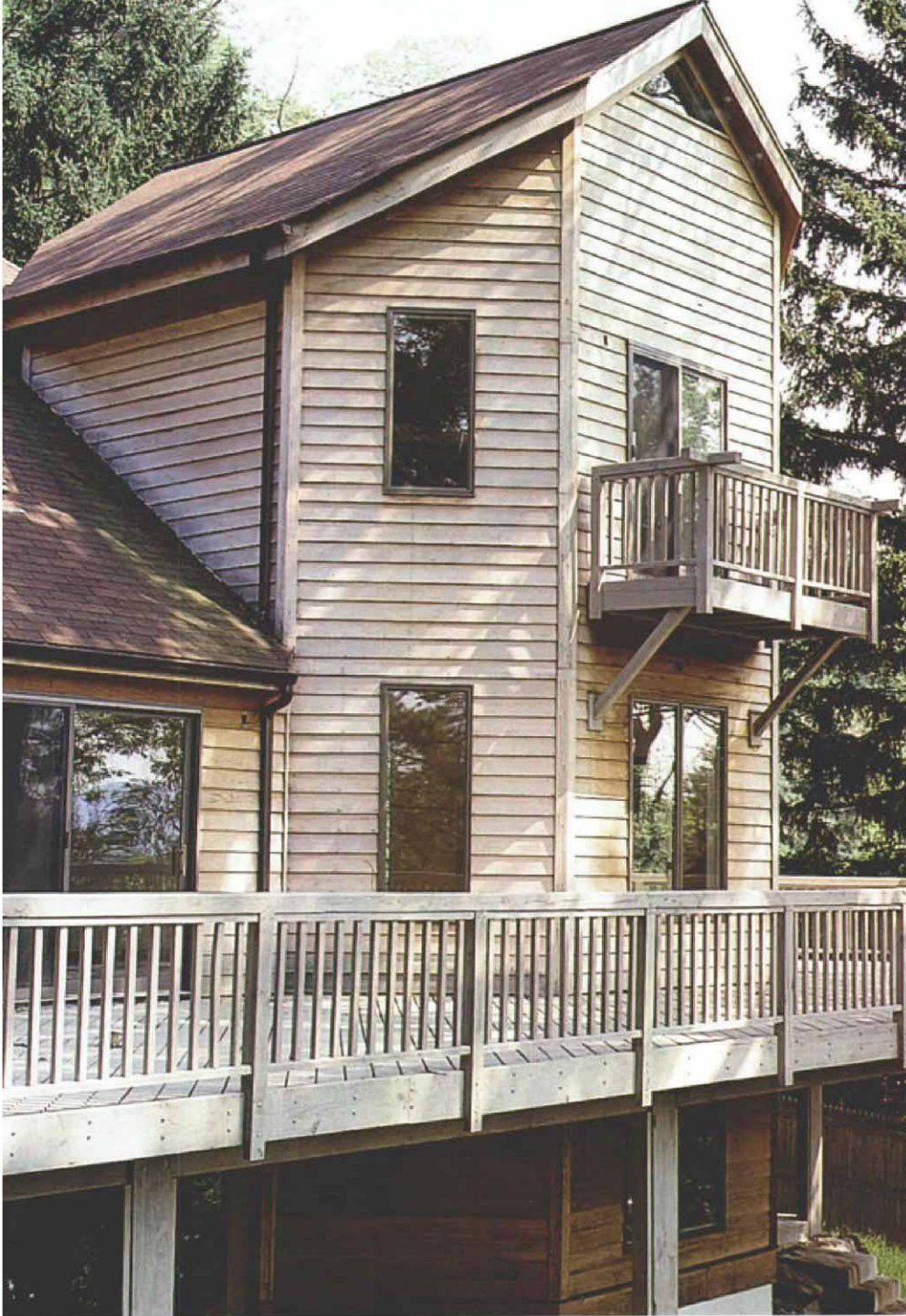
Lopping off the corners. This octagonal room is sheltered by a gable roof that has its four corners lopped off. To find the best way to frame the intersection of the rafters and the sloping, angled eaves walls, the author framed each of the four corners a different way. Photo by Kevin Ireton.
